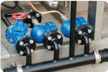
蒸汽疏水阀 Steam Drain Valve
